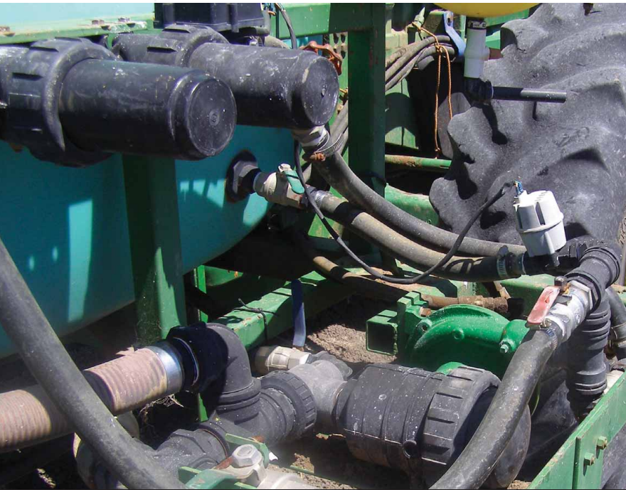
Filter and pump
